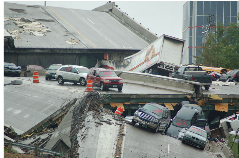
I-35 Bridge Collapse - Minnesota
